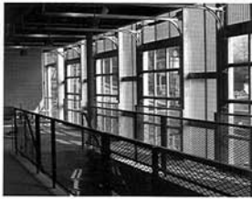
Clockwise from top left: A boiler addition clad in recycled corrugated glass marks the Pittsburgh Glass Center, which reuses a 1920s car dealership. The building is heated in part by recovering waste heat from glass processing. Lights for the gallery space adjust to its occupancy level. Windows that operate like garage doors air the space in warm weather.
