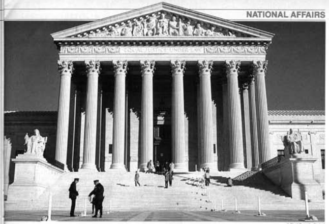
Supreme Court Building: 'A fairly monumental change in the way the government does business'
