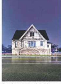
The abandoned houses left behind have been taken down by the thousands. For a while, Detroit couldn't pay for services such as the garbage. With a charter budget crisis, the city has been forced to raise taxes and ending most programs. Some workers have been laid off, and many of those who remain are on furlough.
